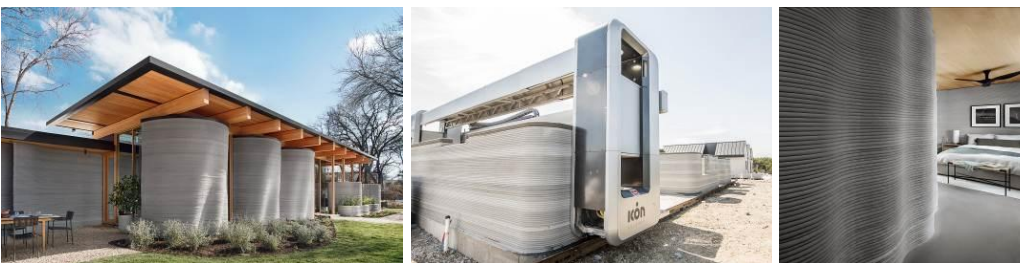
Figure 3. Companies ICON and LAKE FLATO built a 3D printed house Zero in Austin, Texas, 2022 [5]
