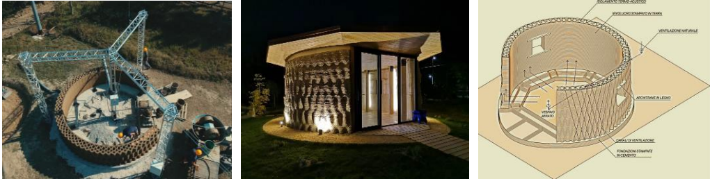
Figure 2. First 3D house printed with soil material, “Gaia”, 2018 [3]
