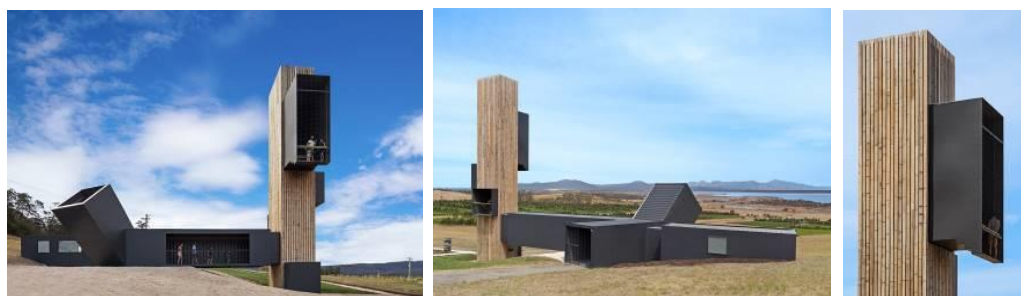
Фиг. 8. Devil's Corner Cellar Door, Apslawn [4].
