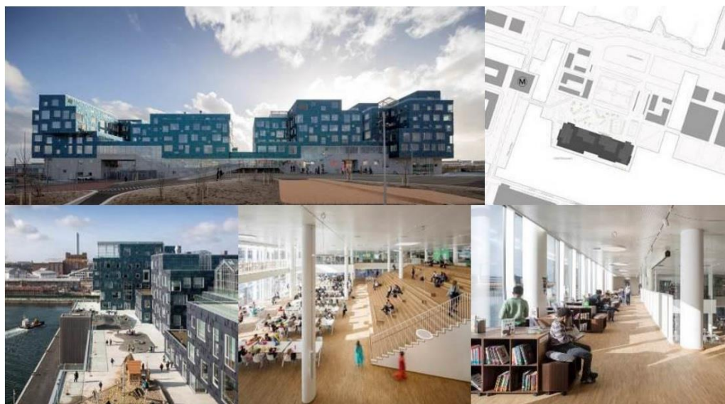
Фиг. 1. Copenhagen International School Nordhavn, Copenhagen, Denmark. Арх. C.F. Møller. Източник: https://www.archdaily.com/879152/copenhagen-international-school-nordhavn-cf-moller
