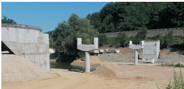
Figure 1. The Graovo bridge construction site, Stationary km 1+302,25 [4]
