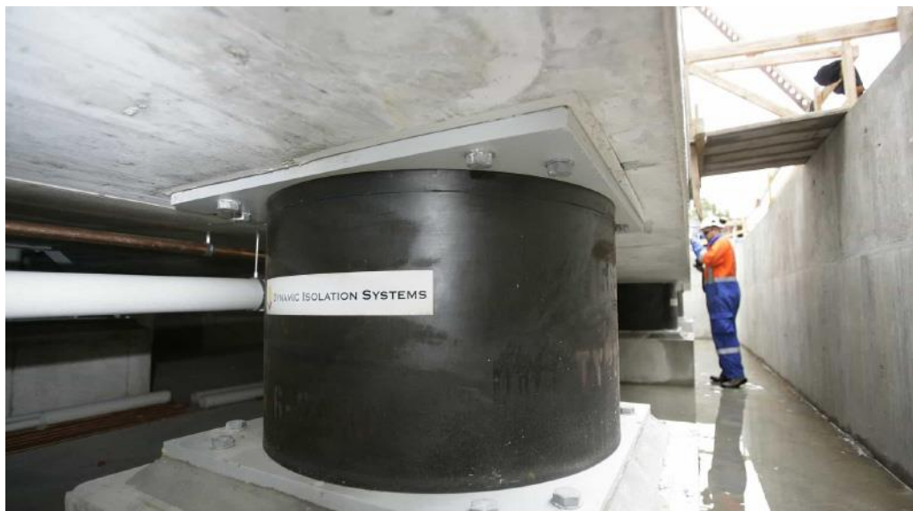
Фиг. 3. Сеизмичен изолатор, Robinson Seismic Limited Company. Източник: https://www.robinsonseismic.com/seismic-isolator
