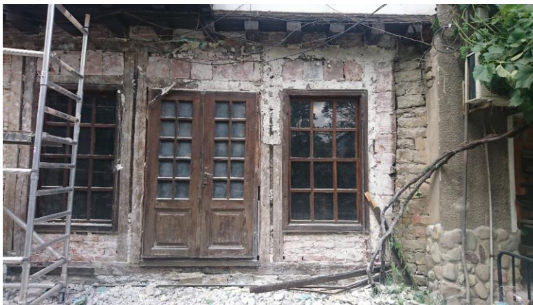
Figure 3. The current state of the main facade
