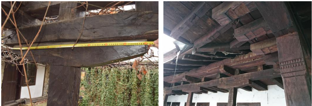
Figure 6. The current state of the beam-column joints
