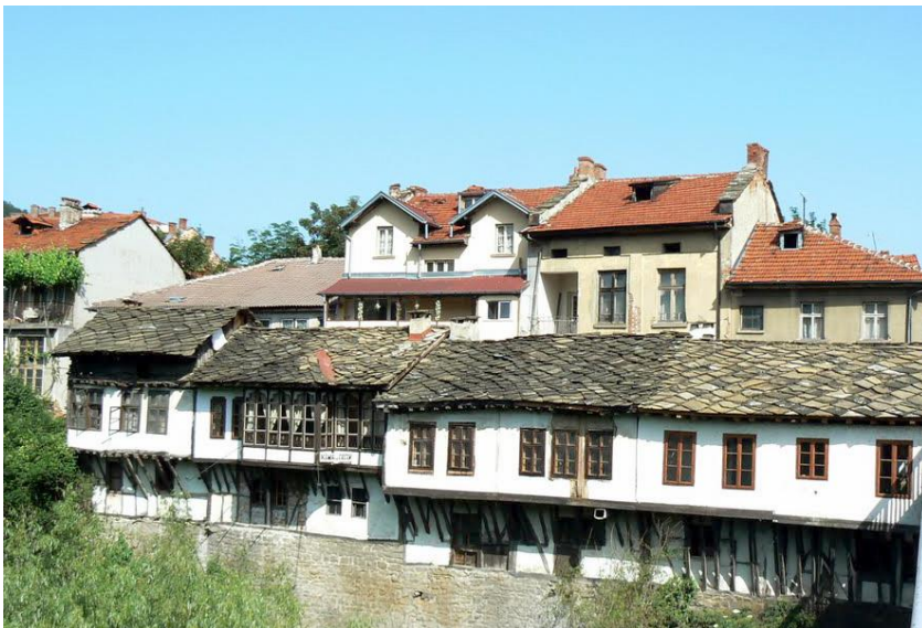
Figure 1. Markov Bridge House Complex, view from the bridge
