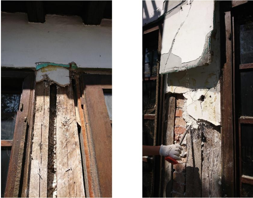
Figure 7. The current state of the timber columns
