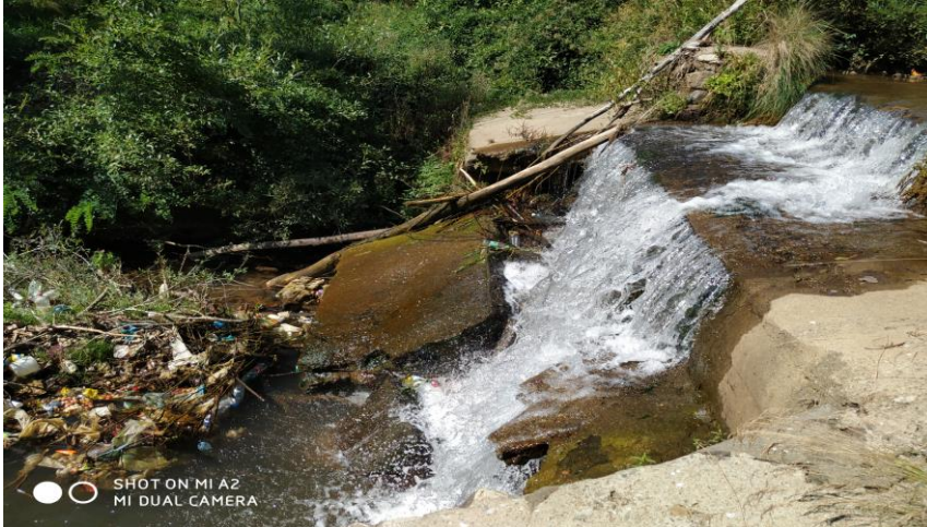
Figure 3. Derogated spillway on the downstream side of the Radovnica Bridge
