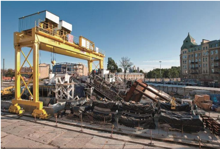
Figure 8. Installation and near surface start of TBM
