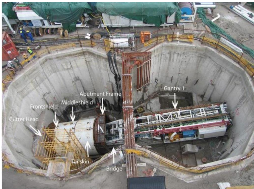
Figure 2. Launching of TBM in the North Shaft
