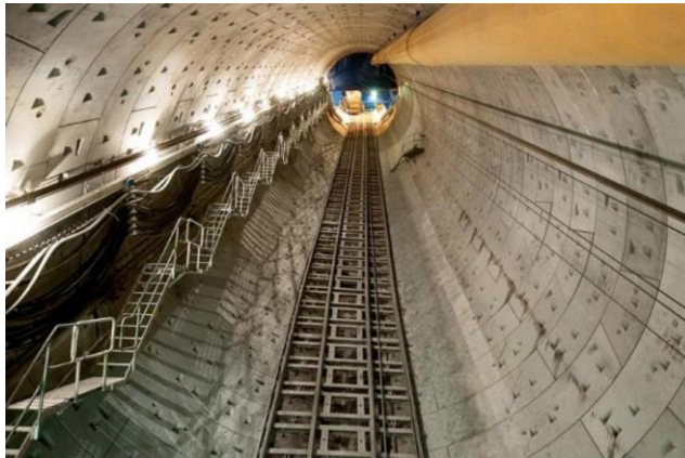
Figure 9. Segmental lining as tunnel support
