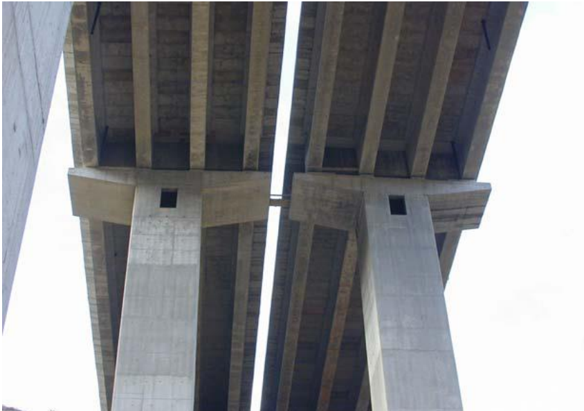
Photo 2. The two branches of the Kavala Bridge
