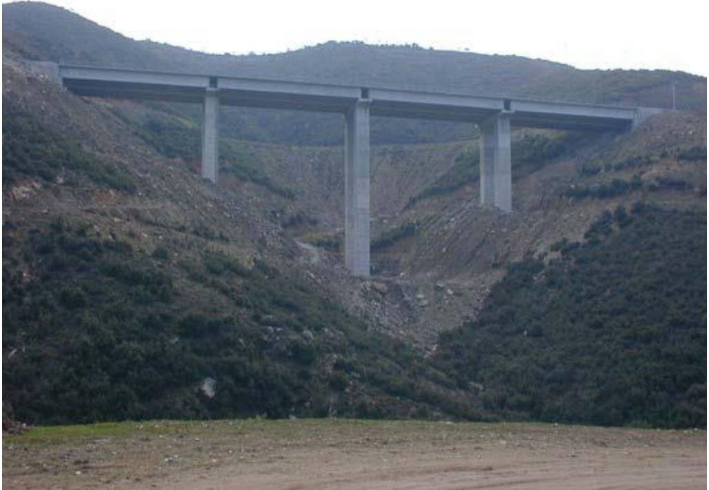
Photo 1. The Kavala Bridge on Egnatia Motorway
