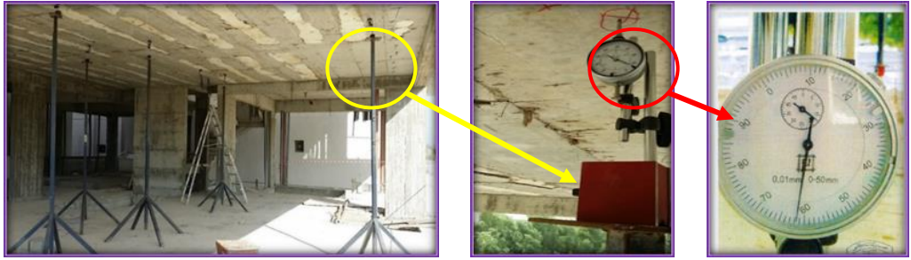
Figure 6. Dial Gauges Installation in F.F.S and Magnetic Holder
