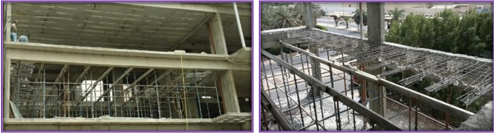
Figure 11. Reinforced concrete slabs after cutting
