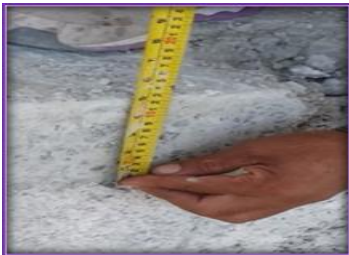
Figure 12. Measuring of thickness of the rib (R1) slab
