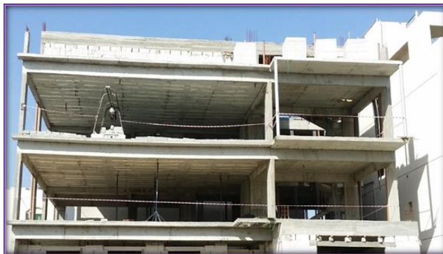
Figure 3. Elevation of building
