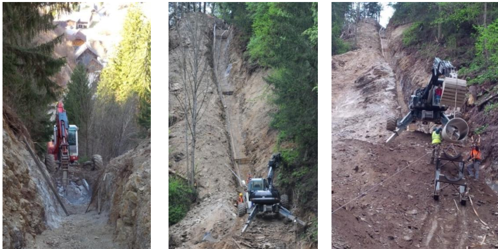
Fig. 10. Penstock placement in the steep section before the powerhouse
