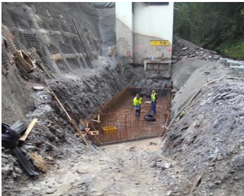
Fig. 5. Collecting tank bottom plate
