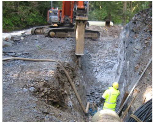
Fig. 6. Penstock placing in the river bed
