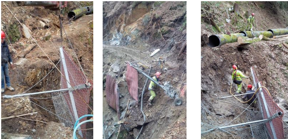
Fig. 8. Installation of slope support system
