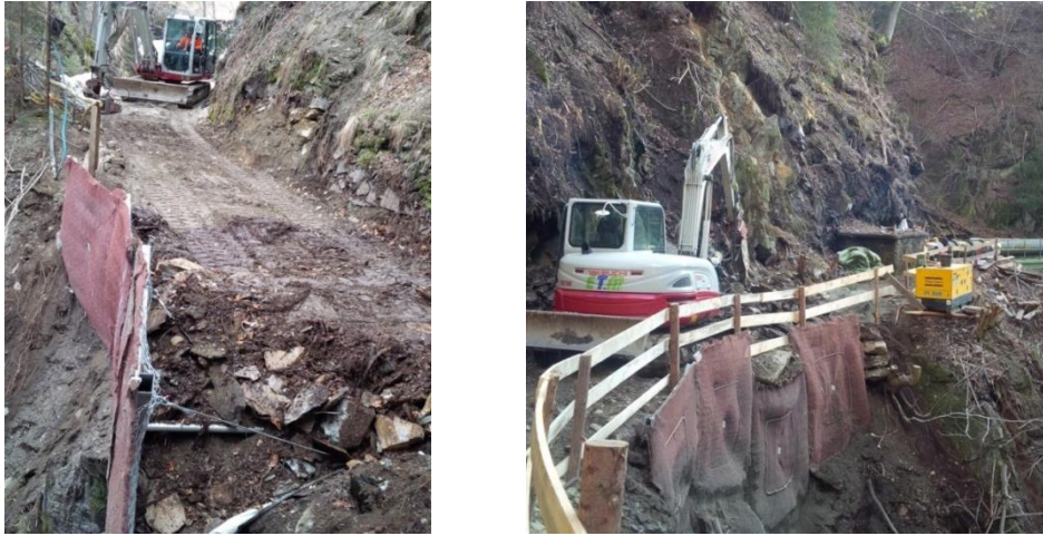
Fig. 9. Access road on top of slope support
