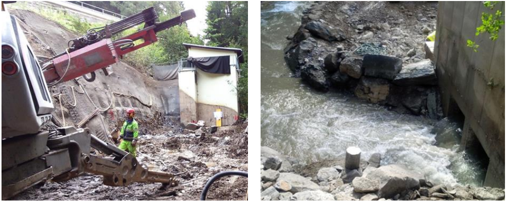
Fig. 4. Slope support and temporary outflow during construction time
