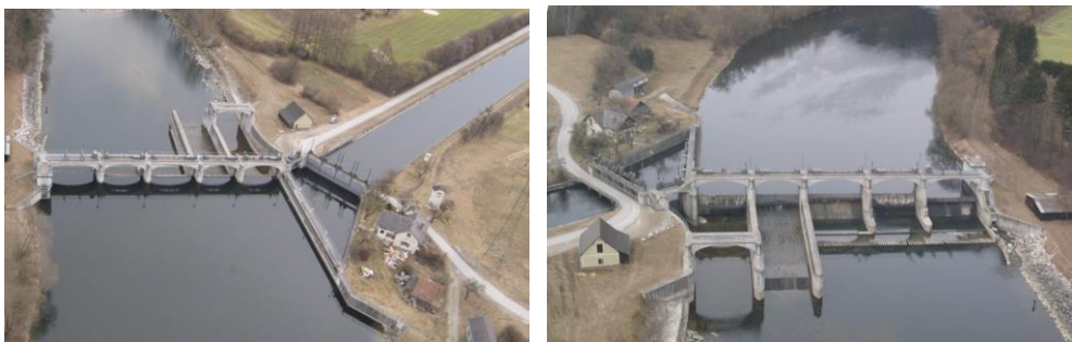
Fig. 2. Upstream and downstream view of the existing Adriach weir with diversion canal (source: VERBUND)
