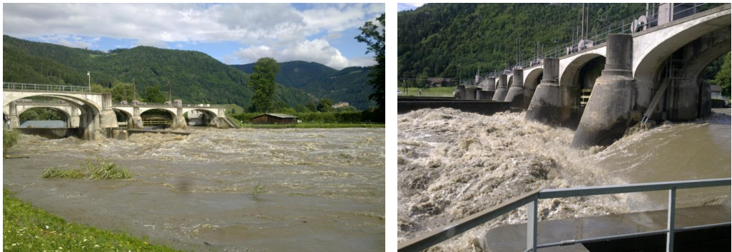
Fig. 4. Downstream region during a Q30-flood water discharge (source: VERBUND)
