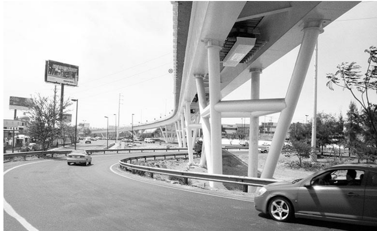
Figure 6. Bridge with TMCS
