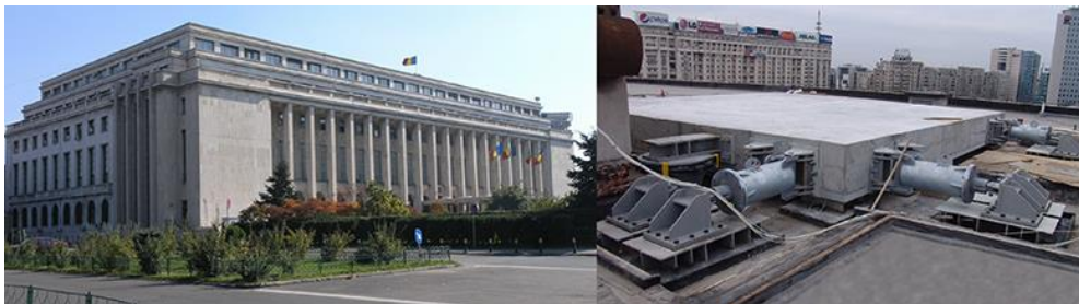
Figure 5. Front view of Palatul Victoria (left side) and TMCS at roof (right side)
