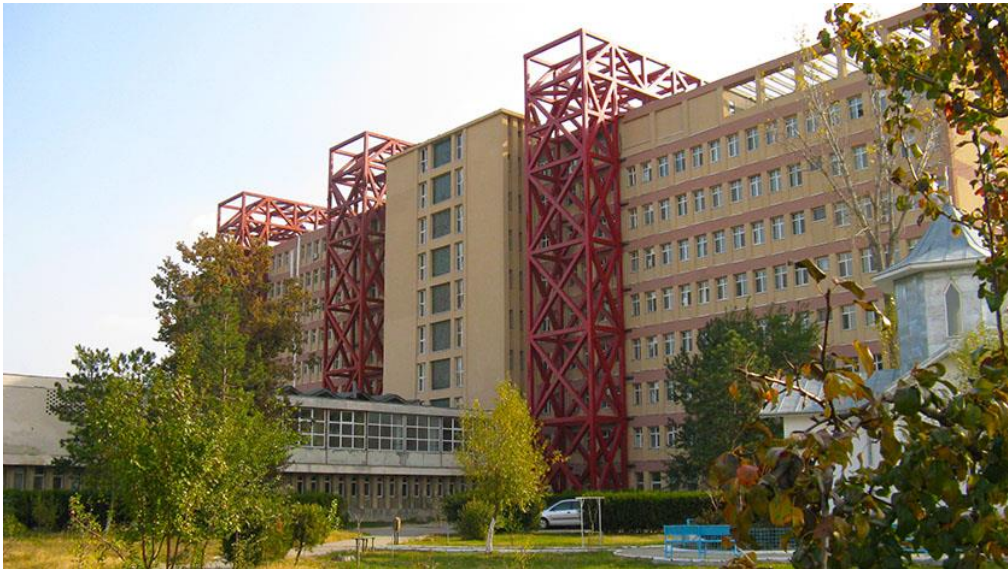
Figure 10. View of the retrofitted hospital
