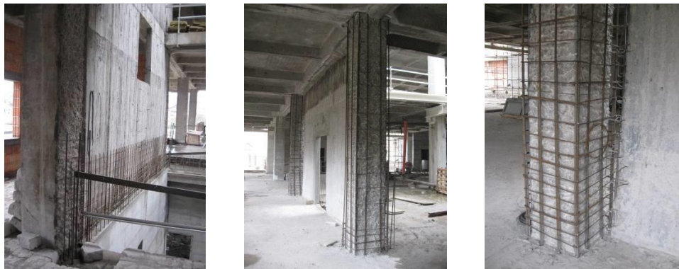
Figure 10. Strengthening the existing RC walls
